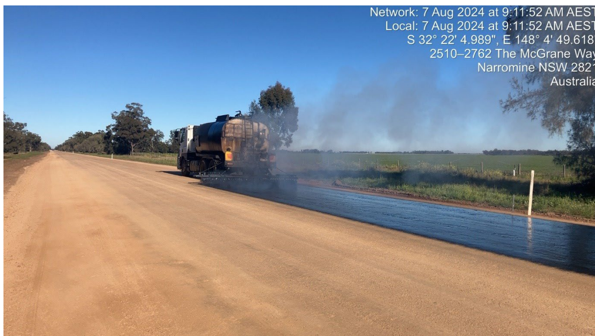
Figure 6: Sealing of Tullamore Road was undertaken in August
