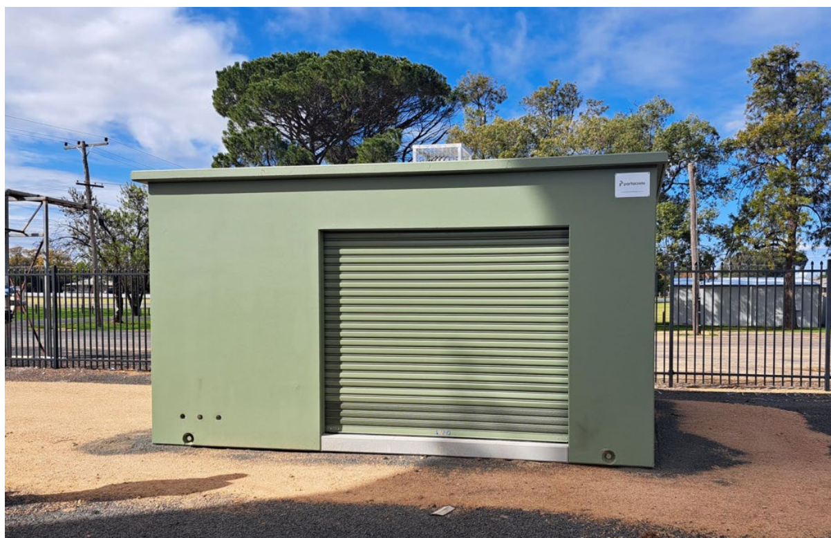
Figure 1: The pump station building on Nymagee Street has been installed.
